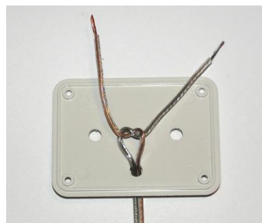
Figure 3.5-2: Power Cord Passed Through the Hole in the Box Lid, and Knotted
